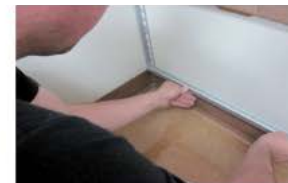
Firmly press the ARTOTRIM-C1 against the wall and add screws to fasten the trim to the wall.
