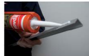
If the tiles need to be cut to the bottom edge of the wall, cut the excess off. Use the ARTOTRIM-C1 and an adhesive caulking to finish.
