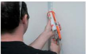
For the tiles that will fit onto trim ARTOTRIM-L1, use a transparent silicone caulking to fasten them into the trim.
