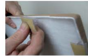
Install ARTOCLIPS-G1 on the side of where the tabs have been cut. The clips facilitate the installation of tiles where the stapler cannot be used.
