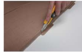
Cut the tabs off the identified files on your plan that will go along the trims, by using a utility knife or scissors.
