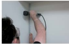
If desired, fasten the trim to the wall by using screws or 12 mm (1/2") staples.
