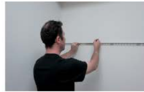
Draw horizontal reference lines on wall or use a laser to level the row of tiles to be installed. Repeat this step for each new row.
