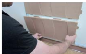
Insert the tile bottom in the ARTOTRIM-C1 and strips in the upper tiles.
