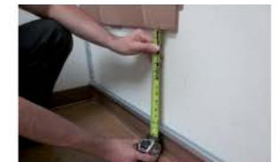
Measure the tile size requirement to insert in the ARTOTRIM-C1.
